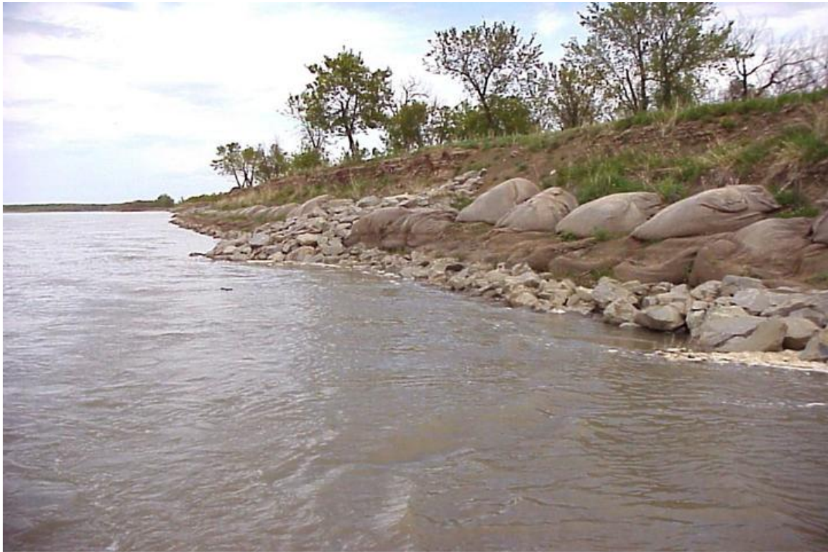
Figure 38. Riprap and bank stabilization restrict river function.
