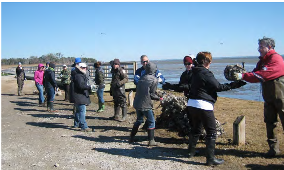
Partners installing an oyster reef in the City of Mobile's Helen Wood Park in south Alabama to provide important aquatic habitat, protect the shoreline from erosion, and act as a natural filter to improve water quality (USFWS).
