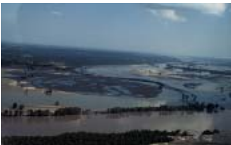
An aerial view of broken levees during the 1993 Missouri River flood.
