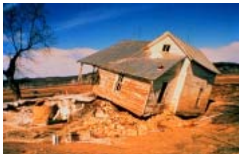
House Destroyed by Flooding During the 1993 Midwest Floods.
