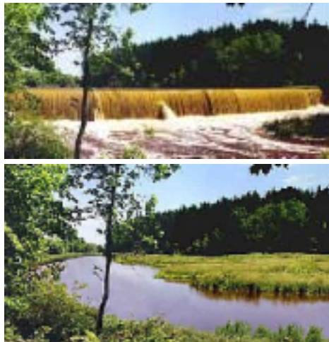
The Franklin Dam on the Sheboygan River, WI before (top) and after (bottom) dam removal. (WIDNR Photos)
