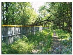
View of a portion of the carp fence designed to prevent Asian carp movements into the CAWS from other waterways during periods of flooding. (Phil Moy Photo)
