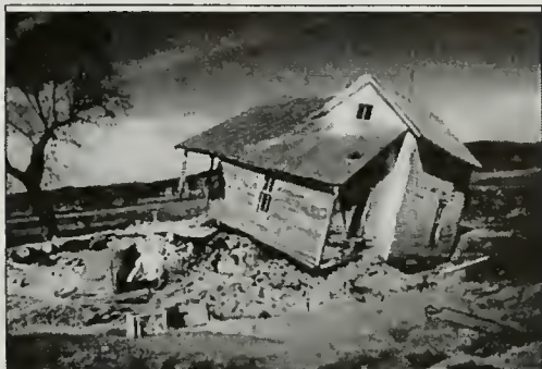
Missouri River floodplain residence destroyed during the 1993 floods.
