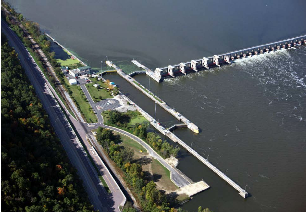
Figure 4. Upper Mississippi River L&D 5 in Minnesota City, Minnesota. USACE photo.
