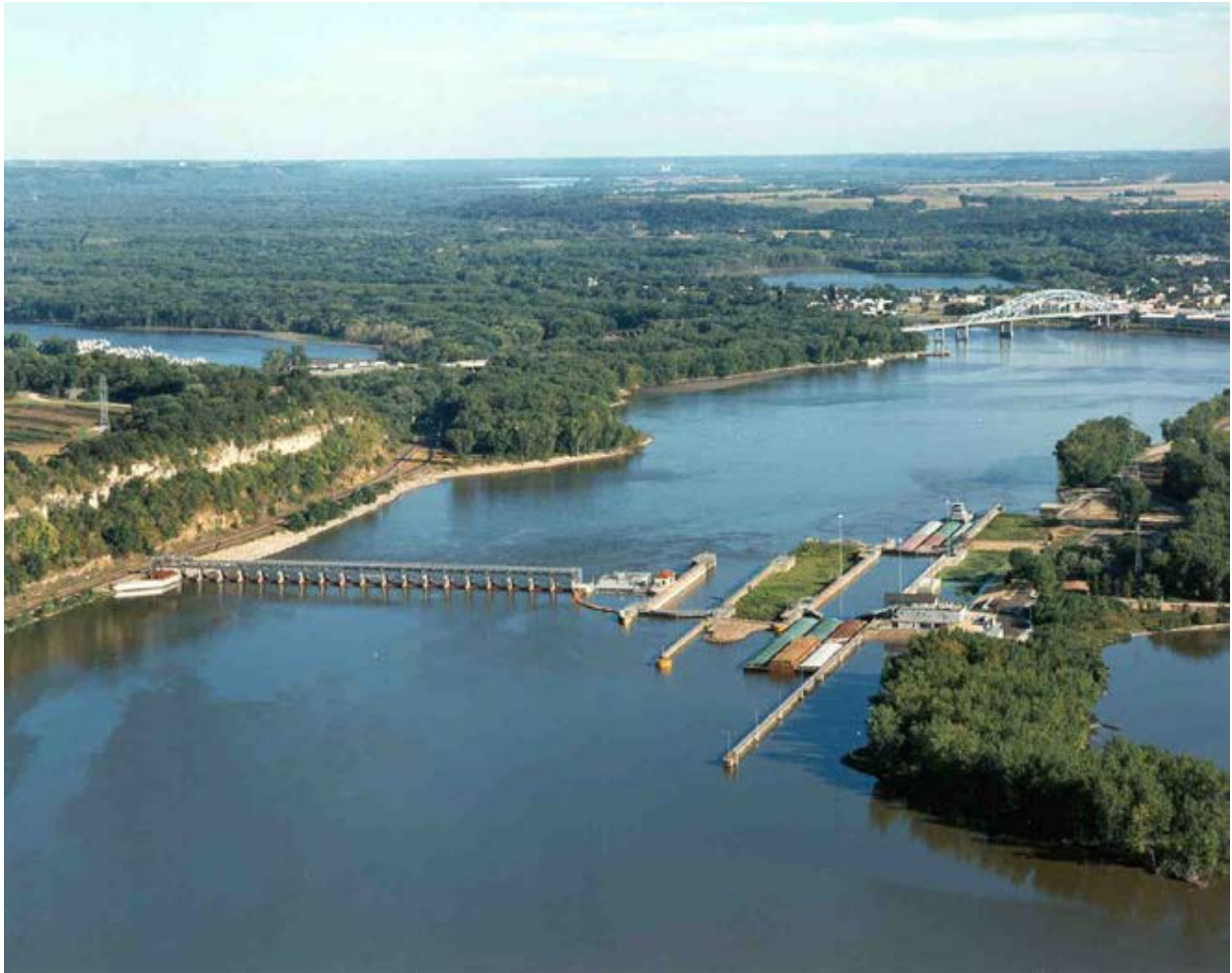
Figure 3. Upper Mississippi River L&D 2 near Hastings Minnesota. USACE photo.
