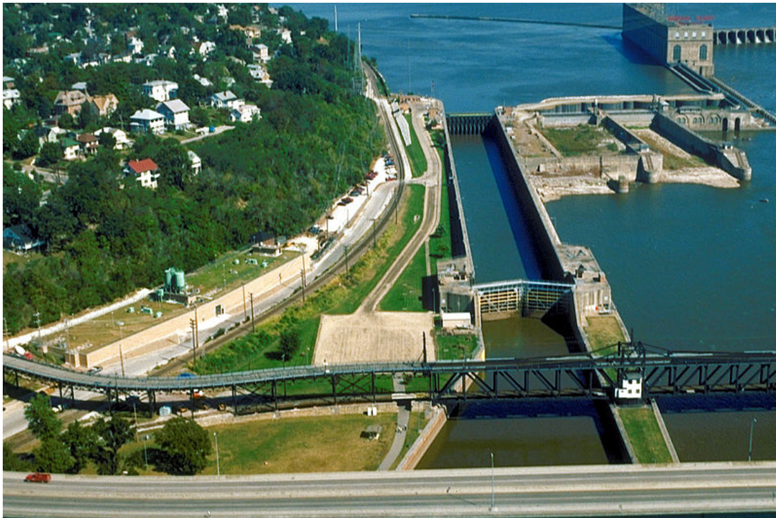
Figure 7. Upper Mississippi River L&D 19 in Keokuk, Iowa. USACE photo
